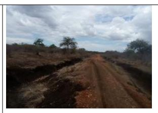
Figure 30: Gulley erosion along the road carriage way
