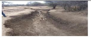
Figure 31: Gulley erosion along the road carriageway
