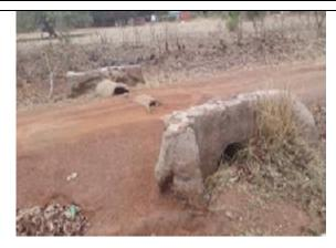
Figure 26: Exposed and broken culverts(km 5.5)
