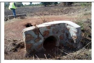
Figure 29: Broken culvert crossing (km 7.4)
