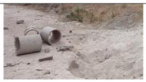
Figure 17: Damaged culverts
