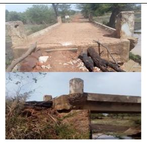
Figure 25: Structurally failed bridge(km16.1)
