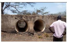
Figure 3: Stream crossing without headwalls
