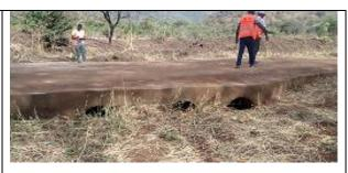
Figure 23: silted vented drift(km 3.6)
