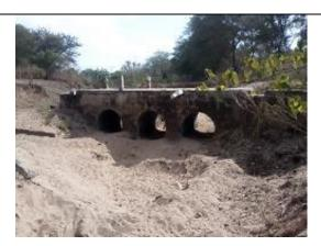
Figure 6: Damaged stream crossing at Robibire stream
