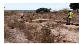
Figure 2:Eroded road section(impassable)
