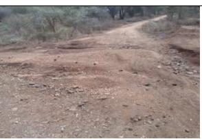
Figure 33: seasonal stream with no drainage structure
