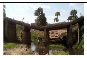
Figure 18: Structurally failed Amua bridge(km 5.0)
