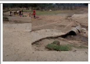
Figure 34: Silted and broken drift(km 12.3)
