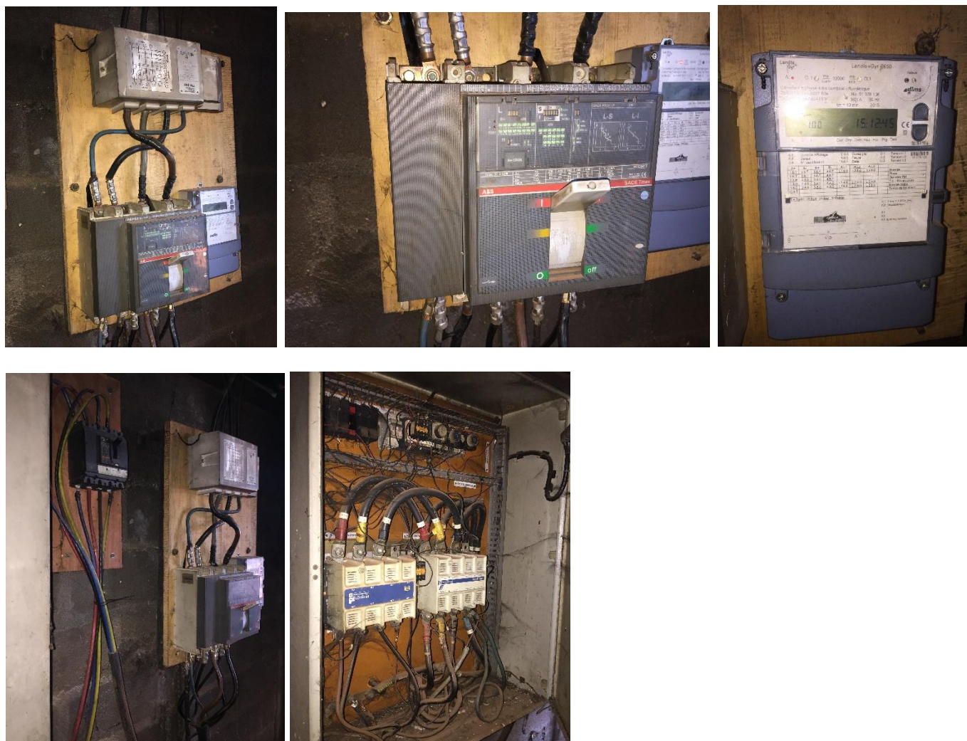
Figure 2. Electrical main switch and distribution board
