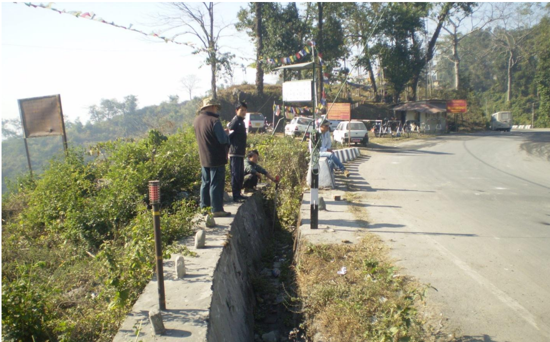
Figure 40: The rain water drains into the landslide crown
