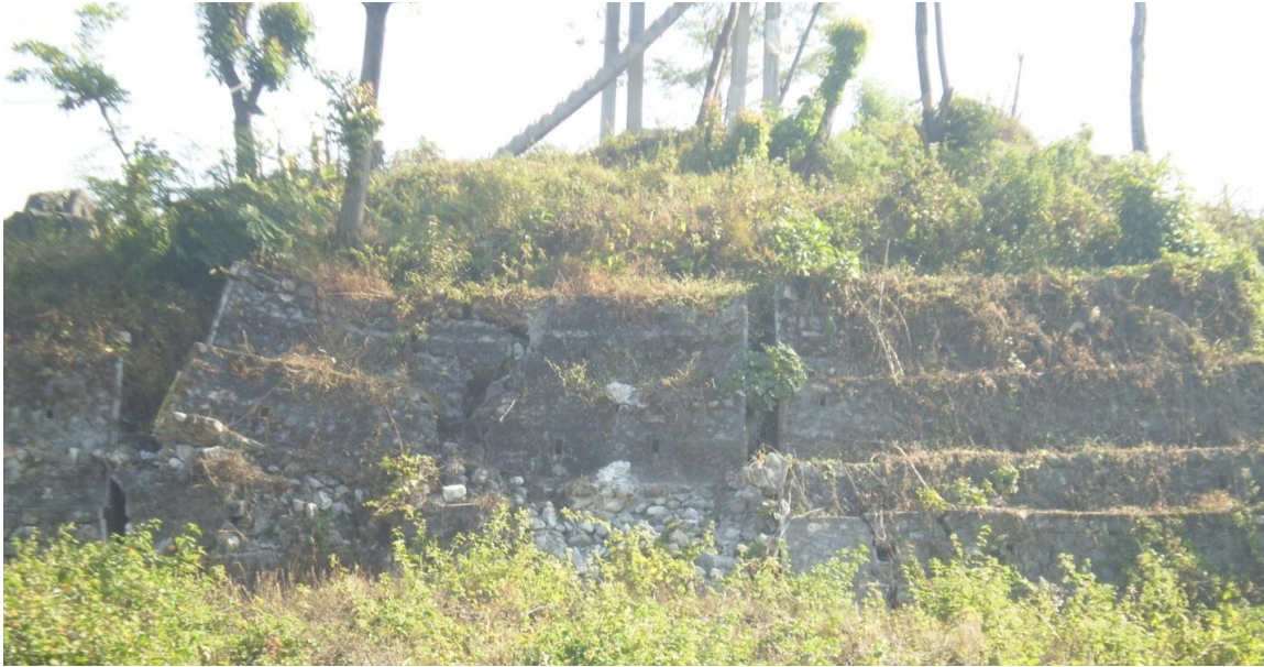
Figure 39: Picture showing the bulged retaining wall with wide open tension cracks
