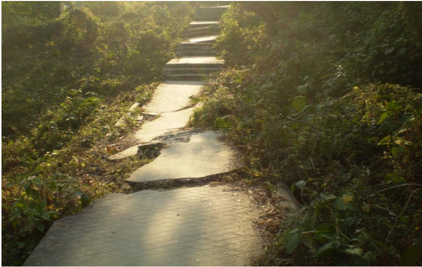
Figure 29: Subsidence of the foot trail leading to old Hospital (MSD) area
