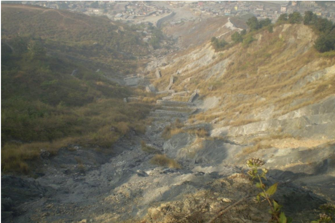
Figure 18: Flexible check dams and retaining structures constructed by Phuentsholing thromde To control the landslide
