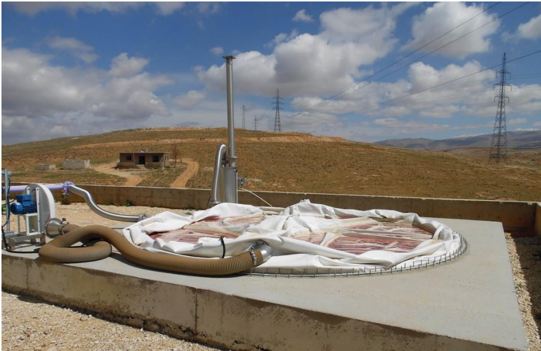
Picture 3. Biogas existing lung
