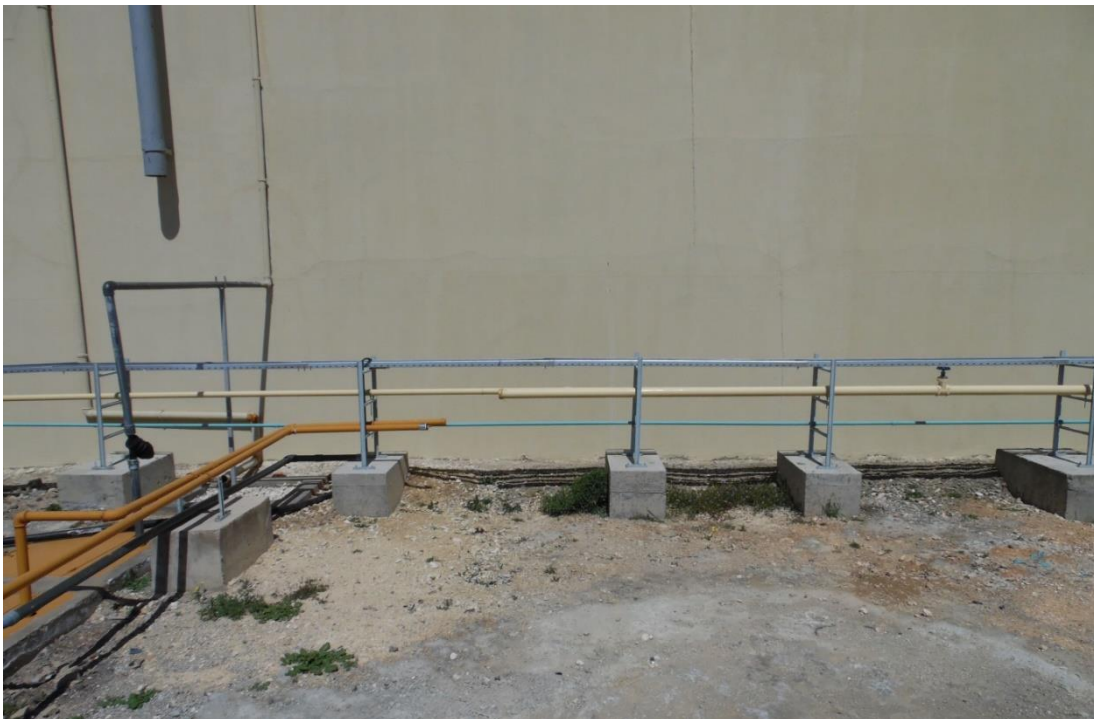
Picture 2. Existing biogas piping system
