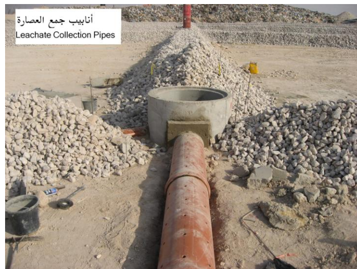
Photo 3: Base sealing system
