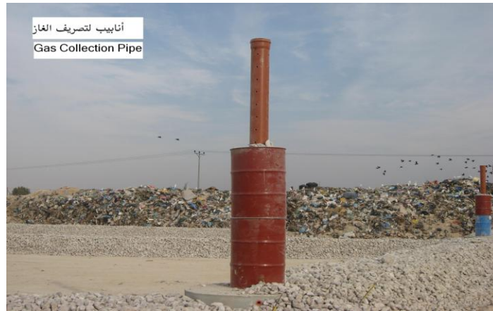
Photo 4: Gas removal pipes
