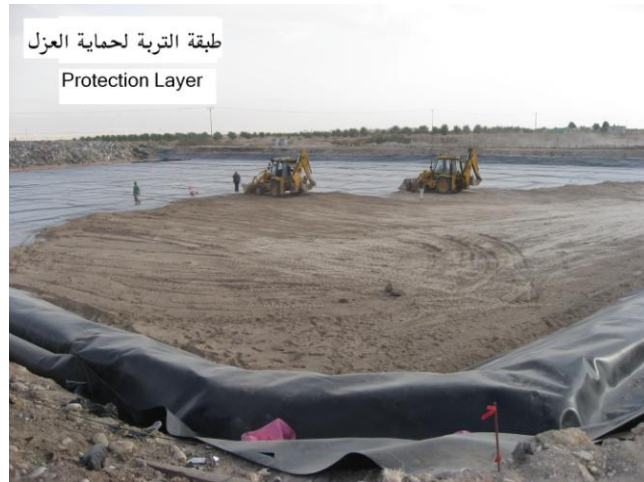
Photo 2: Base sealing system
