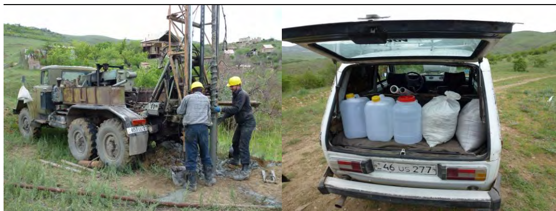
Figure 4.1 Left: The Zil mechanical drill rig in action. Right: Well tubing, clean water, filter gravel and bentonite were transported to the site from Yerevan
