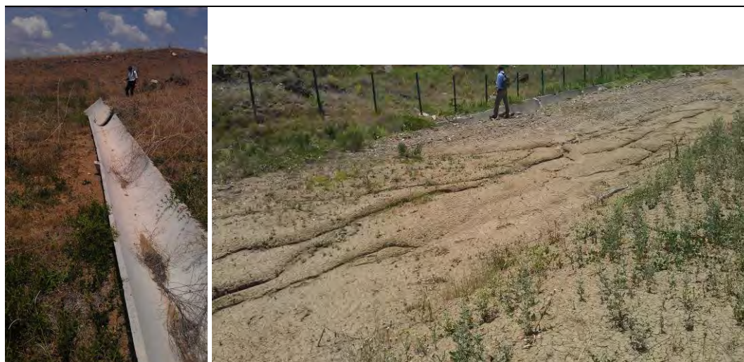
Figure 2.7 Left: Dislocated drainage element. Right: Eroded topcover landfill body
