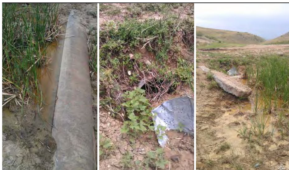
Figure 5.1 Left: The water main preventing the water to flow to the culvert Middle: The blocked culvert Right: Pond 1, the water main, the blocked culvert and the dirt road
