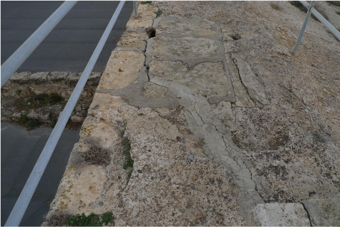
Fig. 35 Cement patches on the crack along the passage way on the top of the external wall of the castle.
