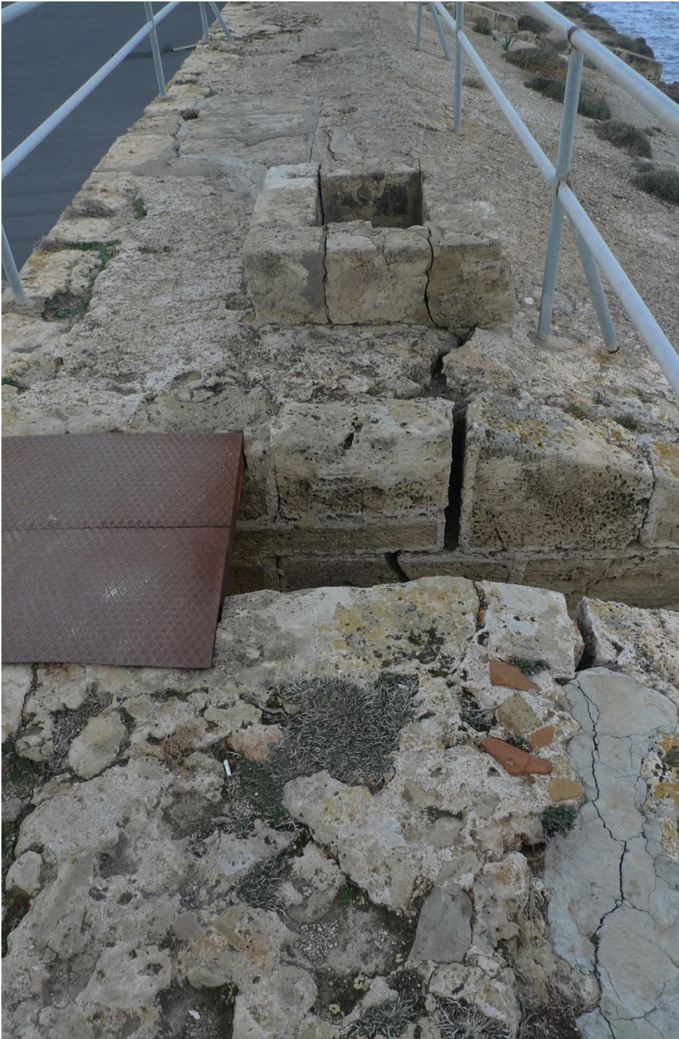
Fig. 15 View of the top of the exterior wall of the castle. The crack runs along the limit between the 1 st and the 2 nd phase of the construction.
