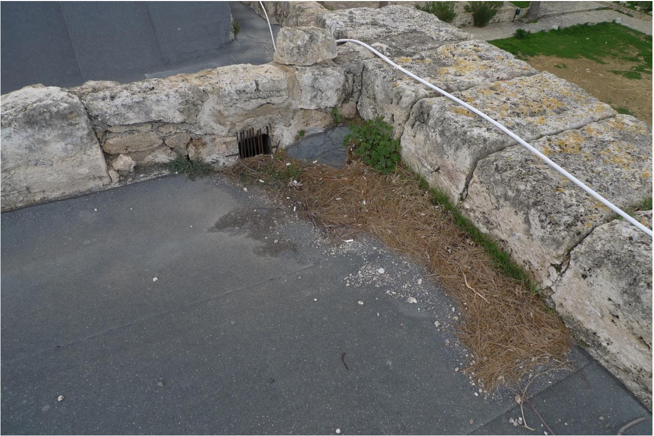
Fig. 16 Detail of the drain of the larger terrace. The membrane doesn't cover the joint between the roof and the walls.
