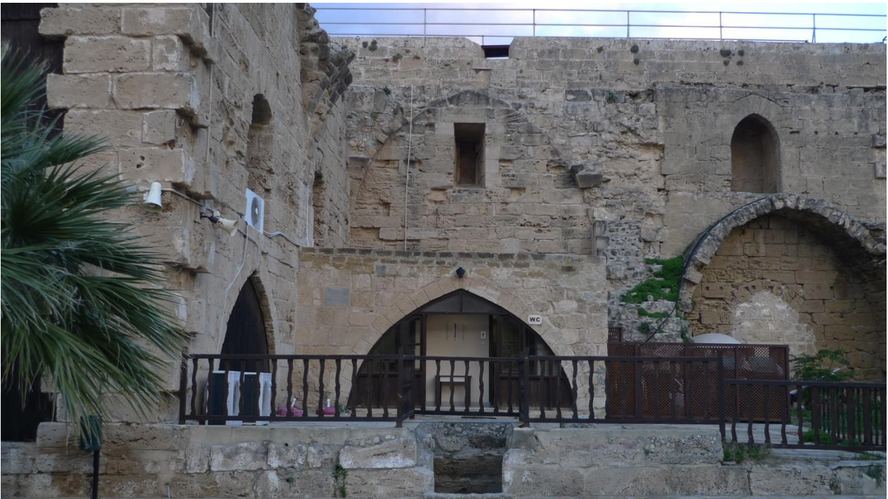
Fig. 2 View of the structures on the South side of the hall with the modern building housing the toilets. Above is visible the original (collapsed) barrel vault.
