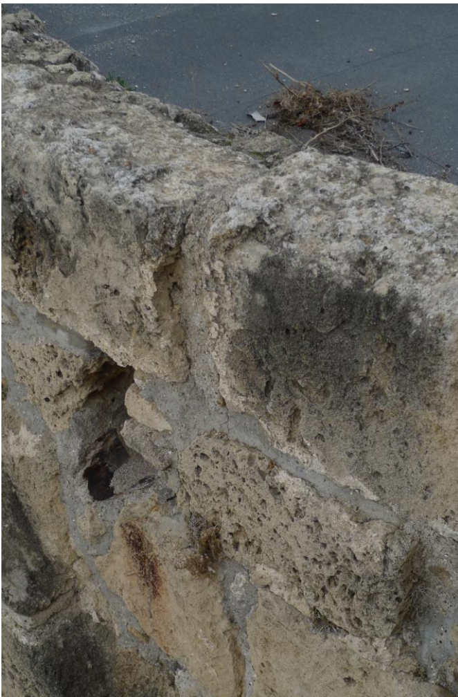
Fig. 36 Water spout originally used for the terrace above the hall. At present unused.
