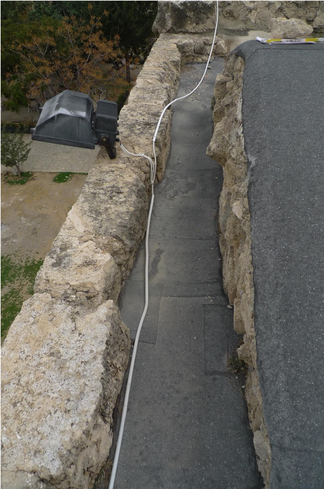
Fig. 18 View towards the Western edge of the roof. On the right – the extrados of the barrel vault covering the hall.
