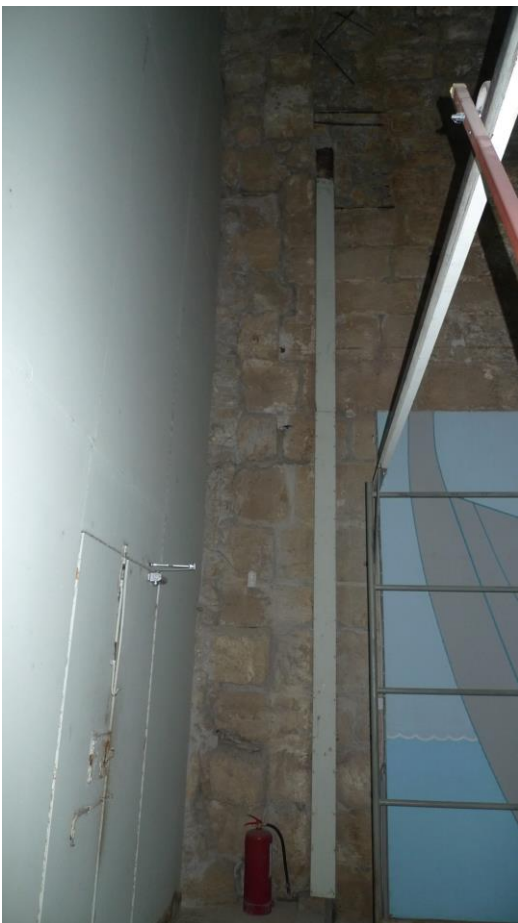
Fig. 28 Downpipe (hidden by an external wooden carter coming from the drains on the roof. There is a concrete patch where the vault was demolished to insert the downpipe.
