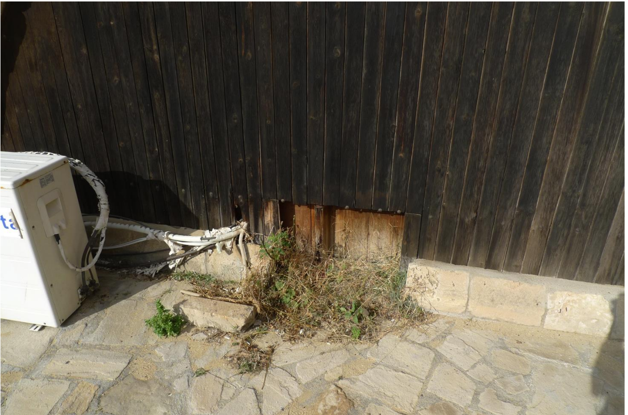
Fig. 26 Damage of the timber cladding and detail of the pipes connecting to interior A/C units
