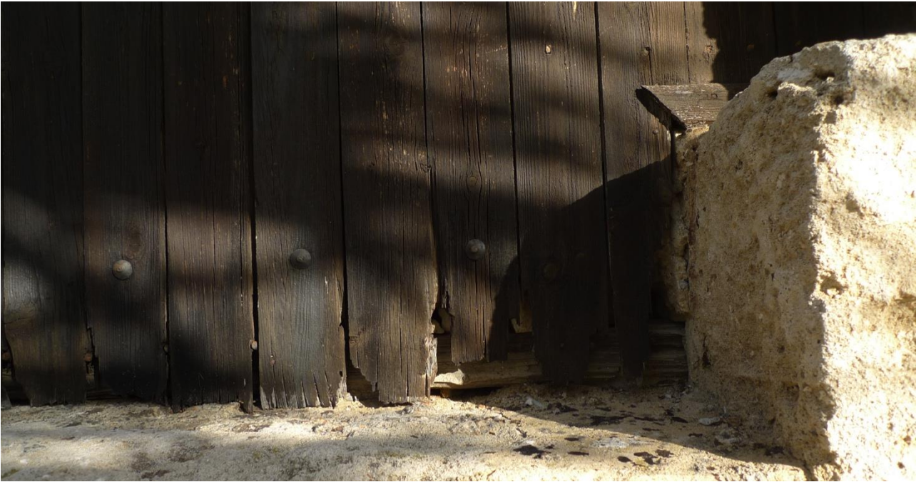
Fig. 29 Bottom side of the timber cladding on the West facade damaged by humidity. The supporting beam is also damaged.
