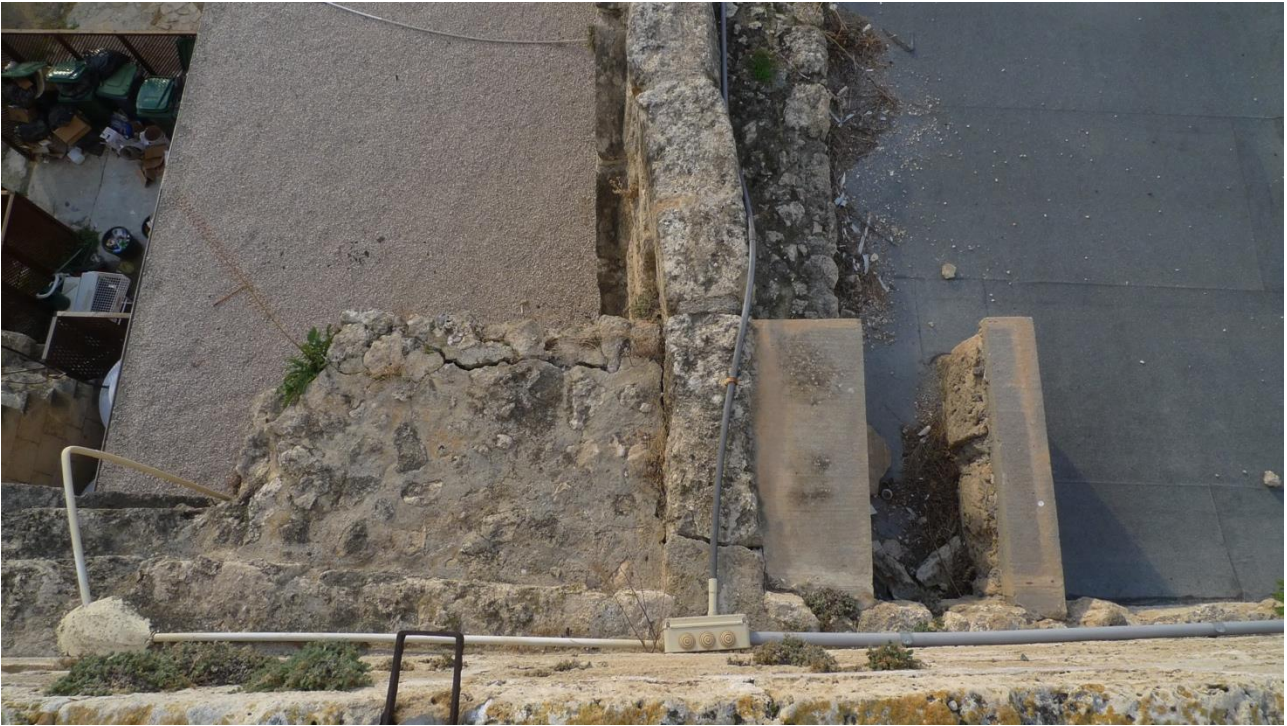
Fig. 12 Detail of the terrace. On the left – remains of a barrel vault with minor crack. On the right – a wall supporting once an external A/C unit (?)
