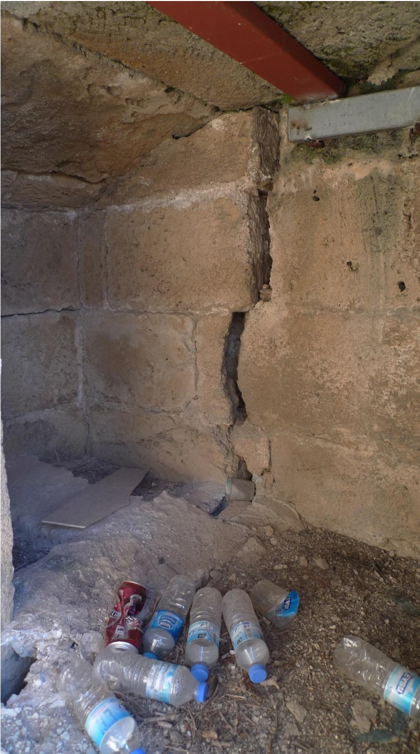
Fig. 31 Crack in a small room under the upper exterior passage way.
