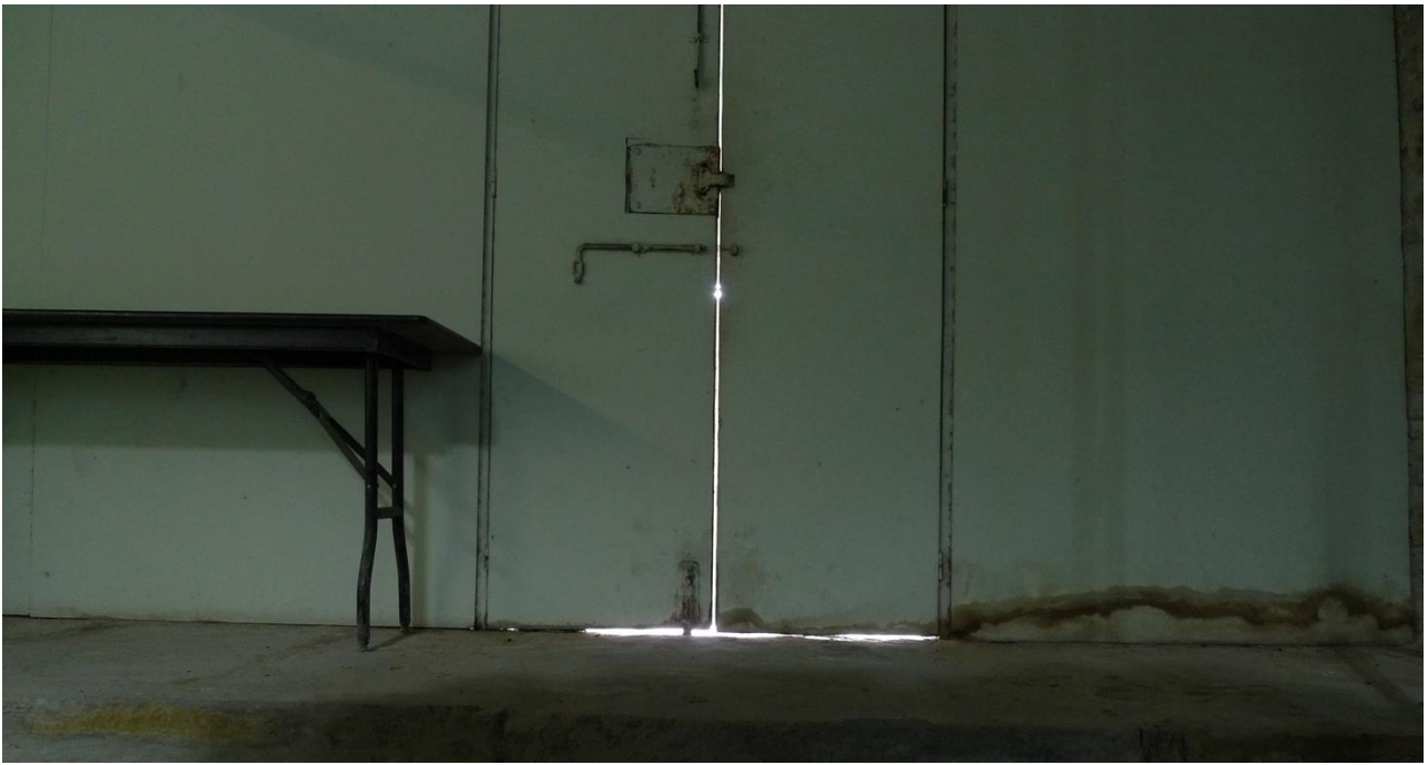
Fig. 27 The entrance door doesn't close hermetically. Damage due to humidity is visible on the interior MDF
