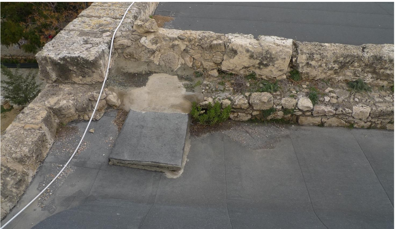
Fig. 17 Detail of the area where the drain of the terrace above the hall is located (hidden by vegetation). The slab is placed on the downpipe.
