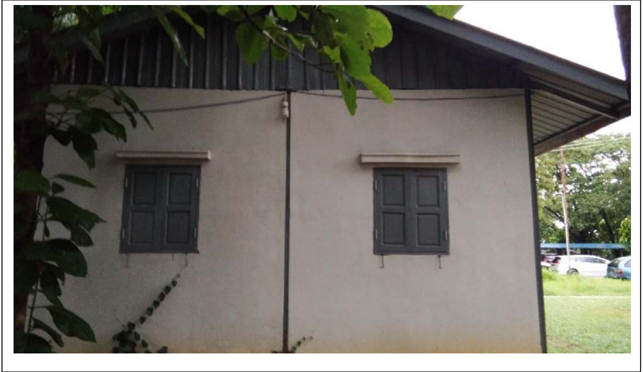
Photo 8 – View from the beside of the building.
