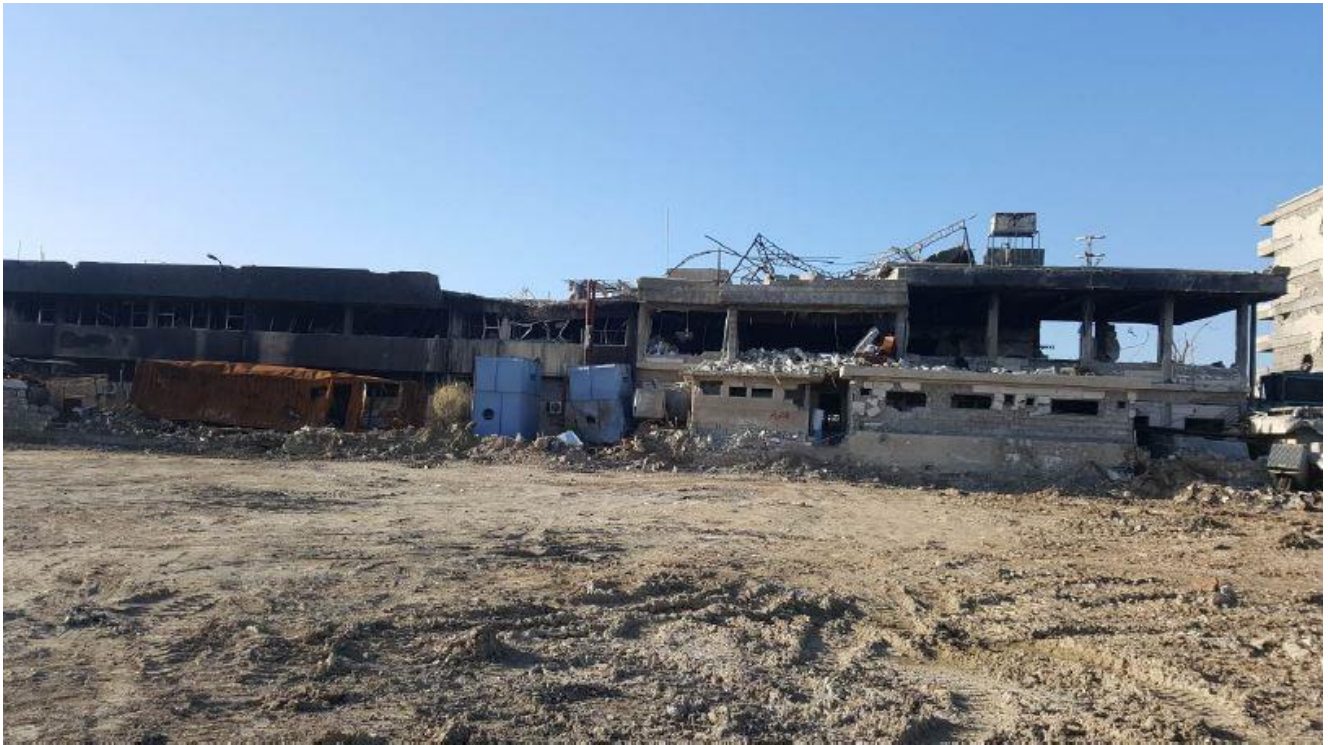
Photo for the Existing Buildings
