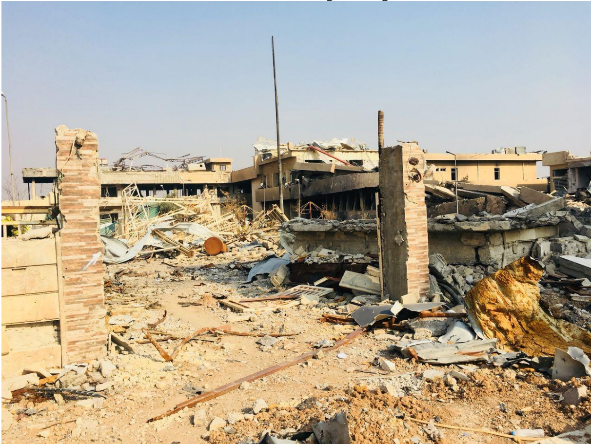
Photos for the Existing Buildings
