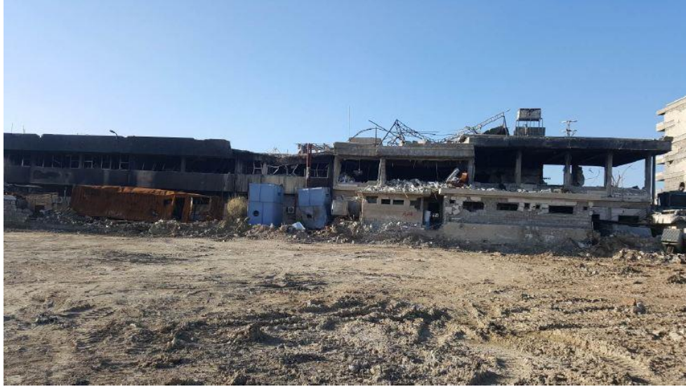
Photo for the Existing Buildings
