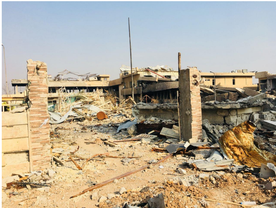
Photos for the Existing Buildings
