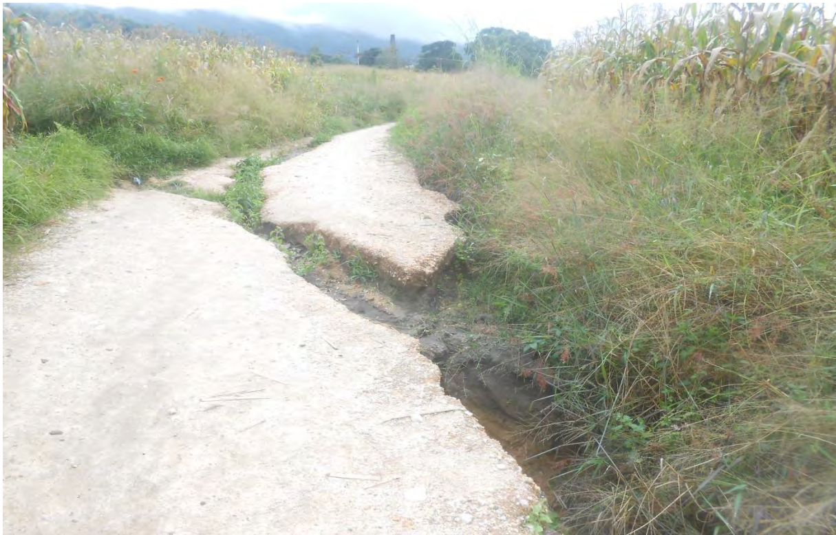
Figure 6 there are two gullies in the vacant stand. The deepest is approximately 1.3m and twenty meters long.
