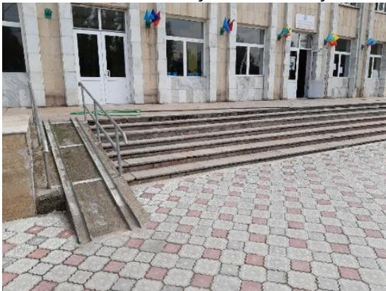
*Photo 3. External staircase with ramp at the main entrance of the building*
