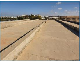
Due to the fire resulting from a direct shell in one of the warehouse halls, which led to excessive damage to the plastering layer, it is necessary to remove the old layer and make another new layer and the subsequent paint work, as shown in photos and detailed in BOQ.
