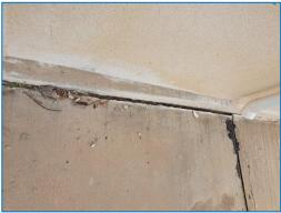
Because of defects in the roof screeding in the building, it will be necessary to supply and laying a bitumen roofing membrane to protect the roof from deteriorating over the time, as detailed in the BOQ.
