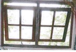
10. Window frame and glasses (600x600) x 2 Steel window frames
