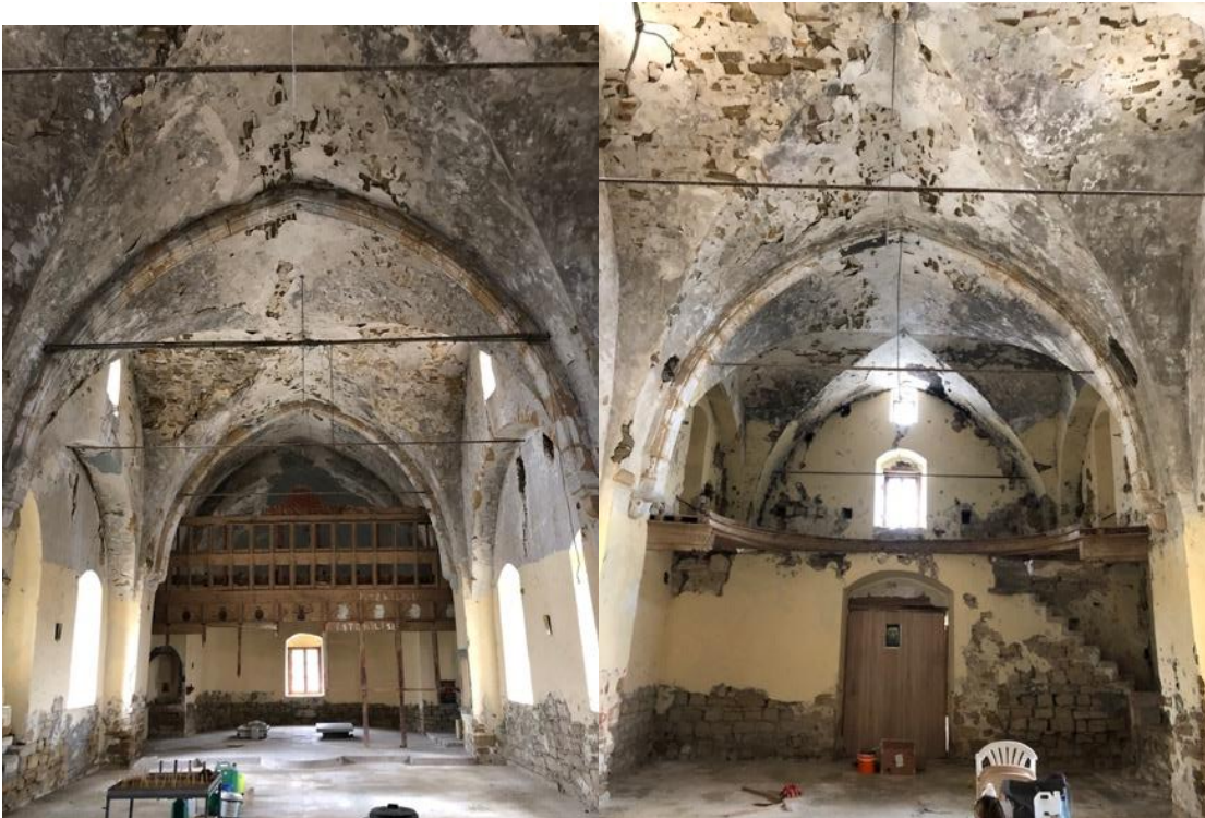
Photos 13 and 14: Roof ceiling: water ingress due to the issues of the roof
