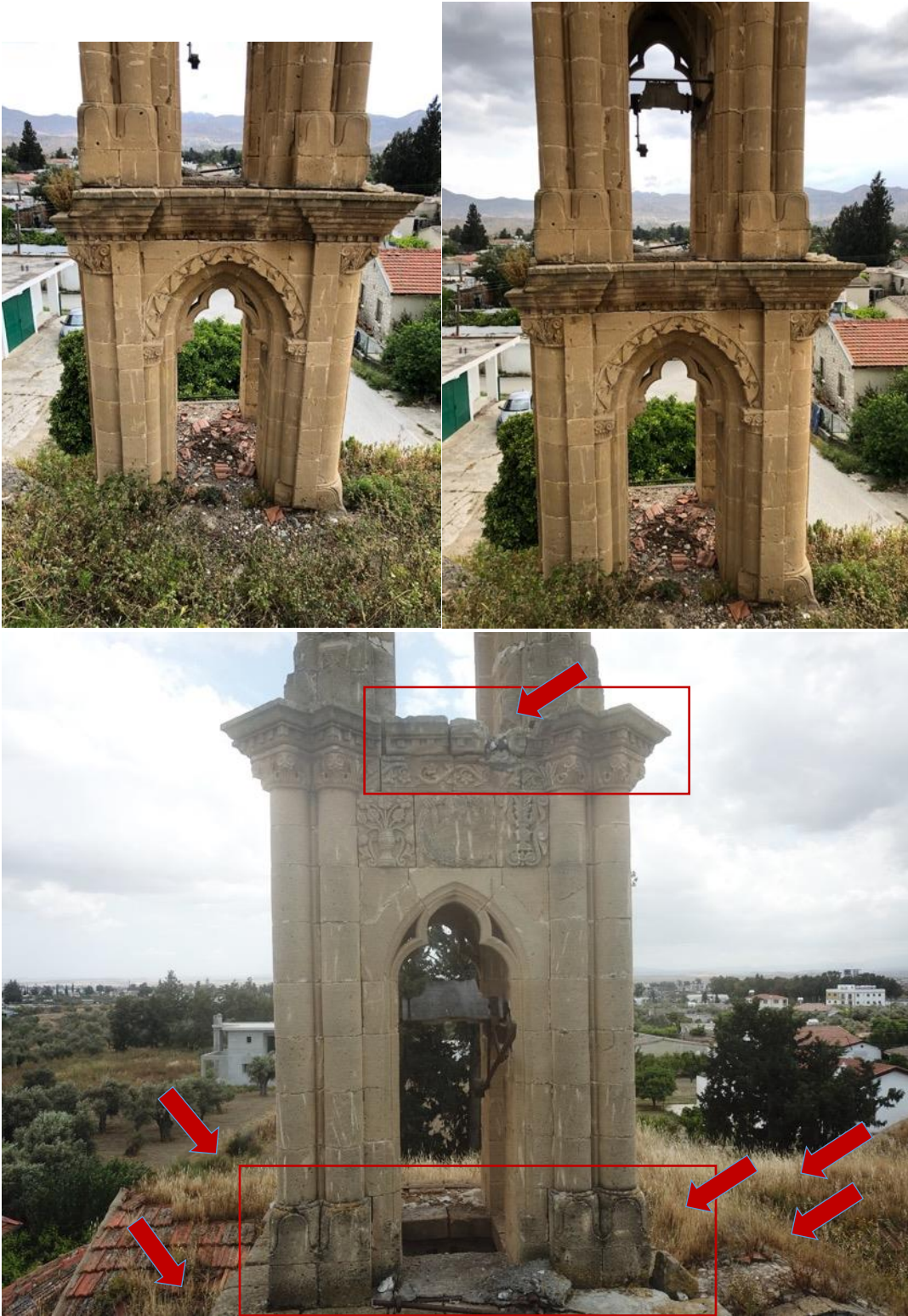
Photos 22,23 and 24 Bell tower: suffering from vegetation, deterioration and loss of materials, erosion of metal elements and inappropriate repairs.
