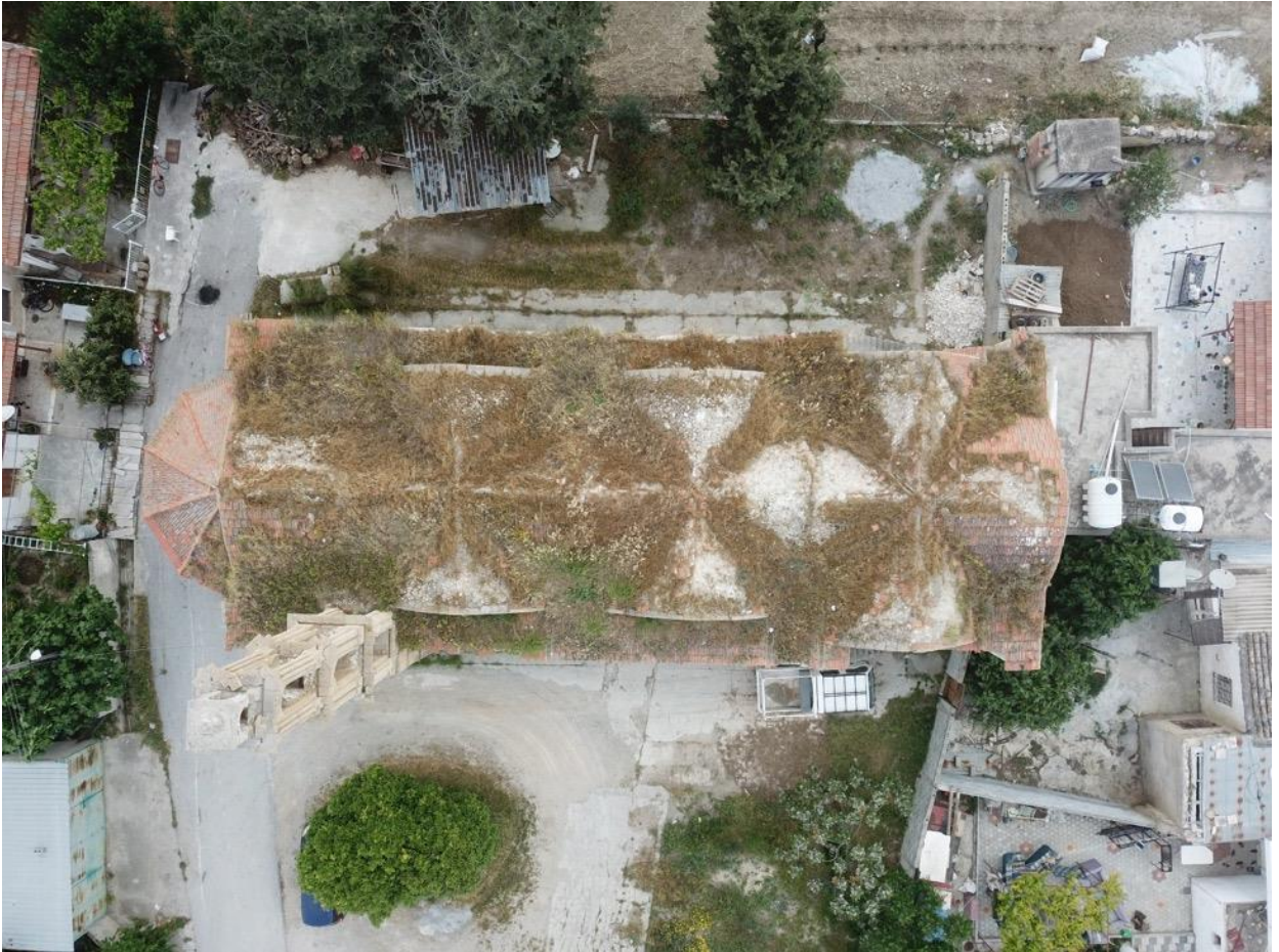
Photo 1: Roof photo: Extensive vegetation, deterioration of the roof mortar and loss of tiles is visible.
