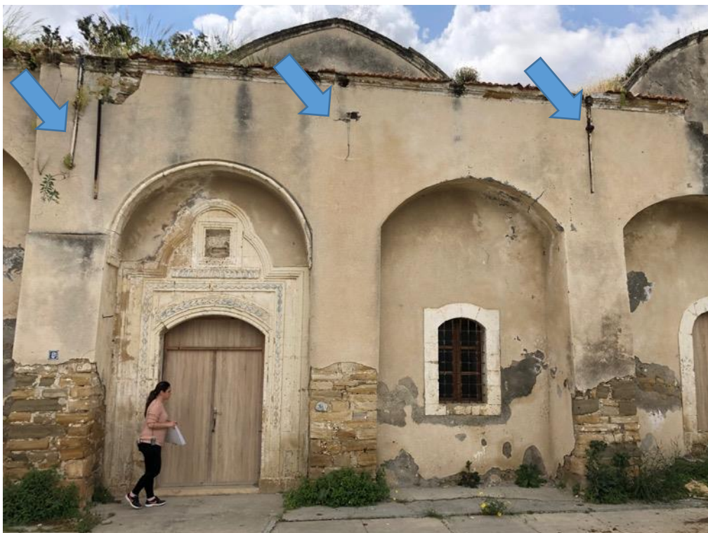
Photos 43 and 44: Metal tie rods / All metal elements should be treated.
