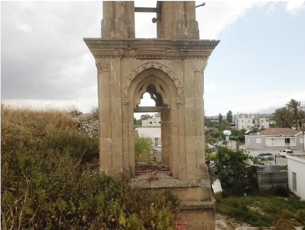
Photos 28 and 29 Bell tower: suffering from vegetation, deterioration and loss of materials, erosion of metal elements and inappropriate repairs.
