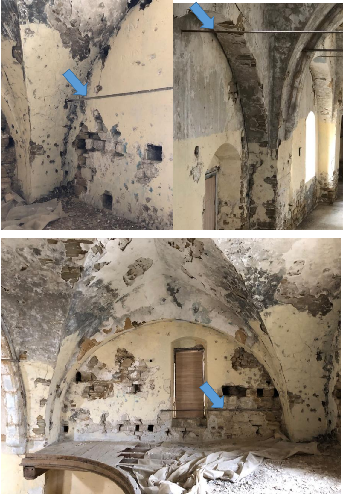
Photos 40,41 and 42: Metal tie rods / All metal elements should be treated.
