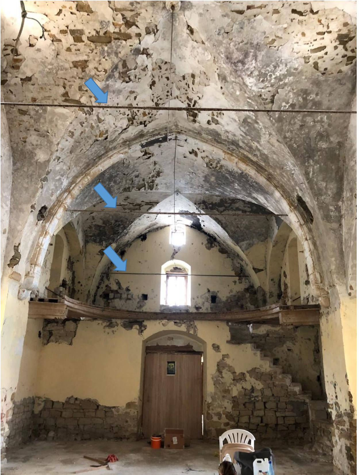
Photo 39: Metal tie rods / All metal elements should be treated.
