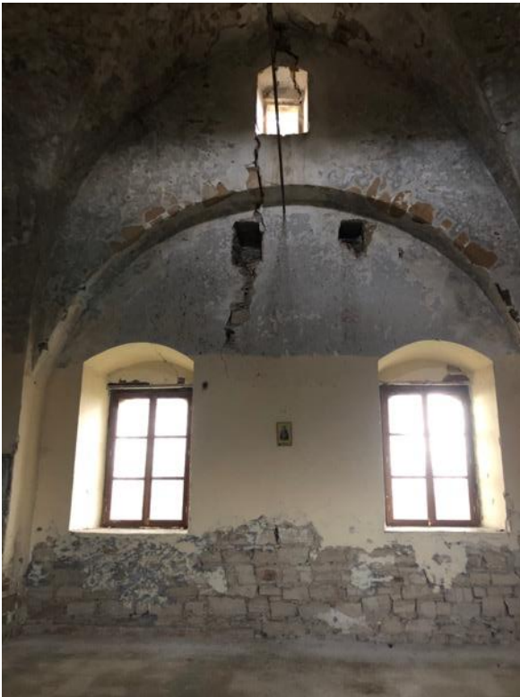
Photo 56.7 and 56.8: Cracks / Indoor
