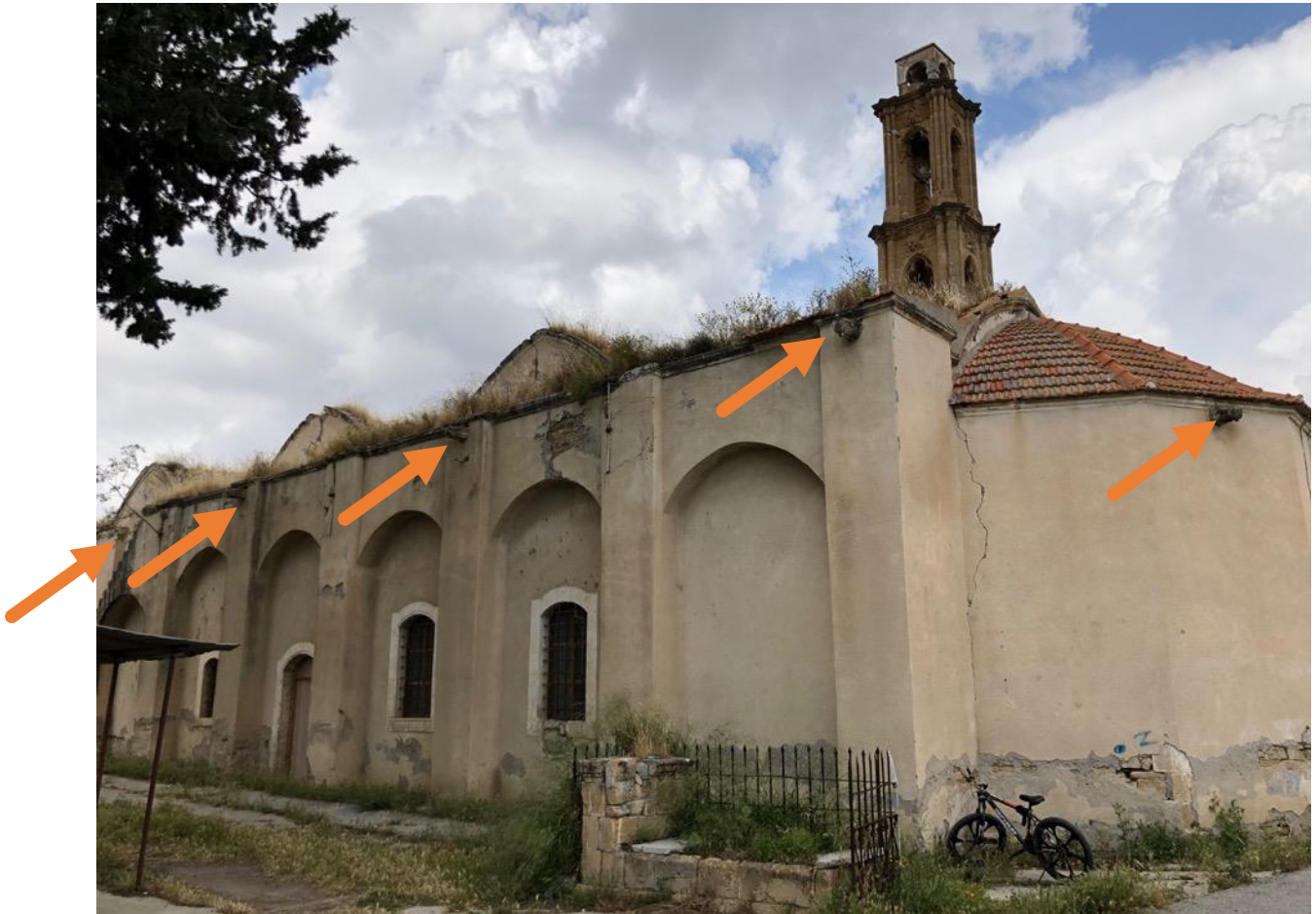
Photo 10: Existing waterspouts/ South facade
