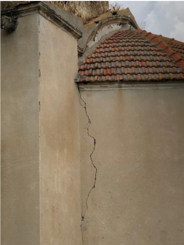
Photo 56.1, 56.2, 56.3, 56.4: Structural cracks to be treated
