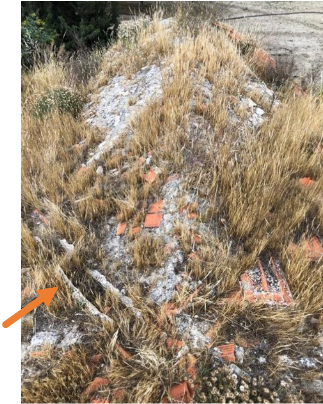
Photos 7 and 8: Roof photos existing drainage system channels are indicated
