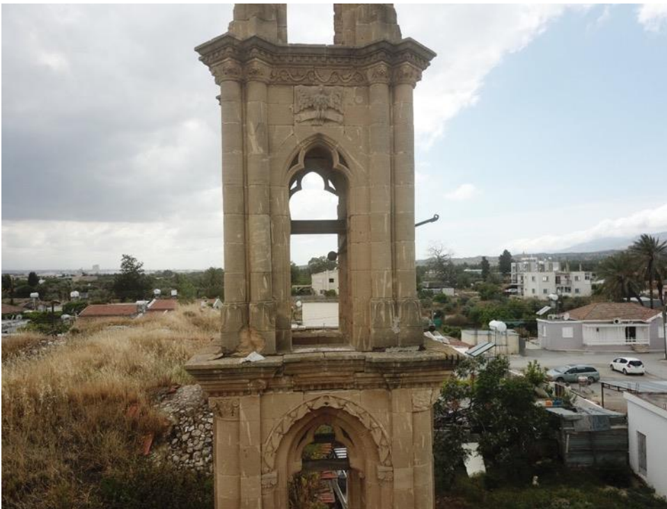
Photos 25 and 26 Bell tower: suffering from vegetation, deterioration and loss of materials, erosion of metal elements and inappropriate repairs.
