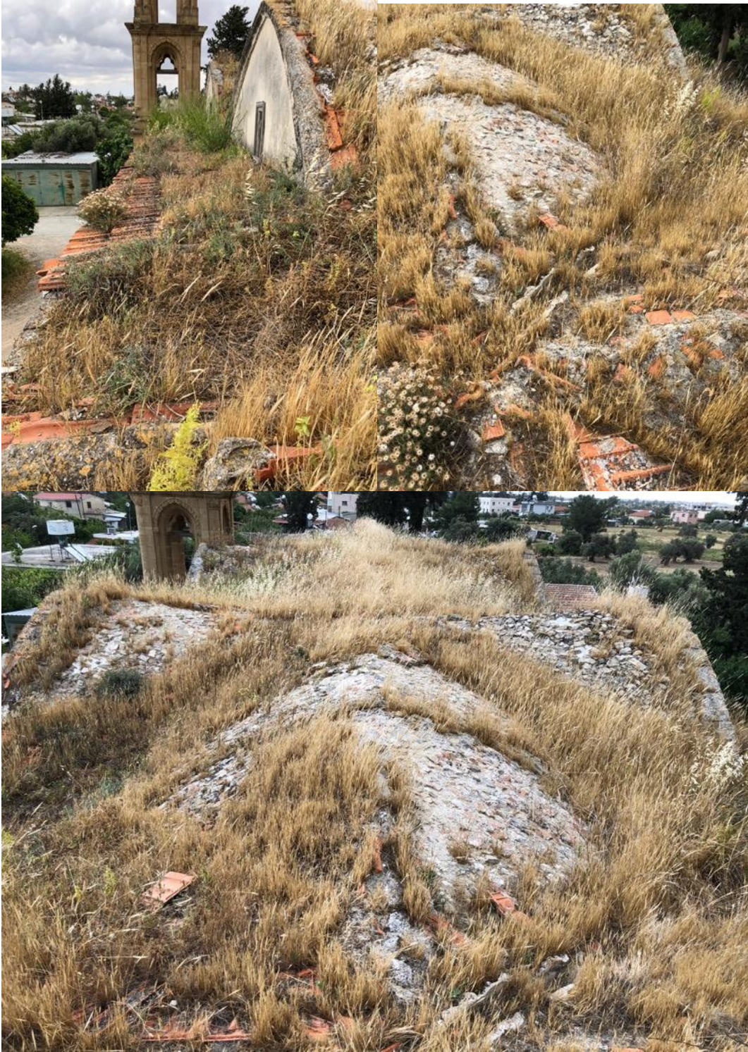
Photos 2, 3 and 4: Roof photos: Extensive vegetation, deterioration of the roof mortar and loss of tiles.
