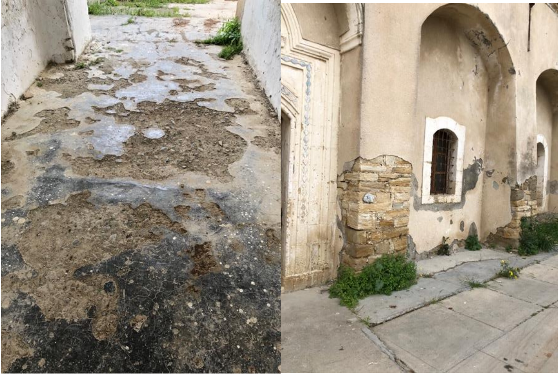
Photo 46 and 47: External concrete floors to be repaired: Narthex area flooring is made of gravel and very thin cement layer on top. Rest of the courtyard is concrete
