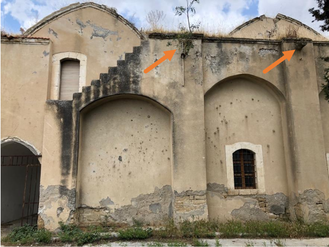
Photo 11: Existing waterspouts/ South facade
