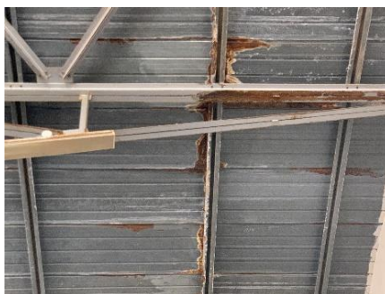
Rust to Metal ceiling and truss
