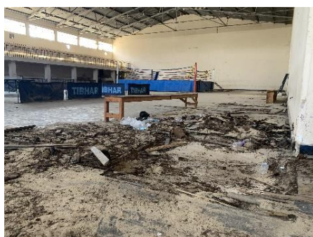
Fracture to wooden floor
