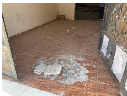
Fracture to ceramic tiles
