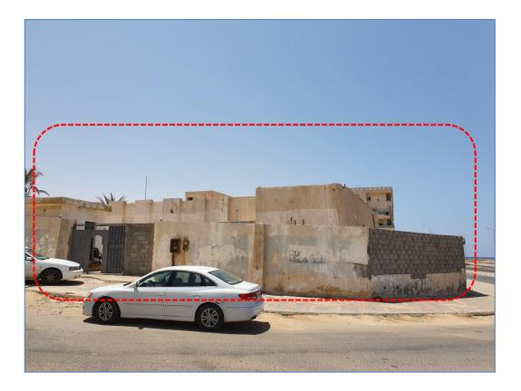
Also, some external walls, parapet and structural elements has suffered many deterioration which needs to be rebuild and rehabilitate similar to the existing as shown in the photos and the BOQ.
