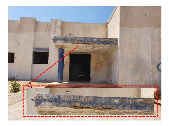
Because of the fire, which led to excessive damage to the plastering layer, it is necessary to remove the old layer and make another new layer and the subsequent paint work, as shown in photos and detailed in BOQ.
