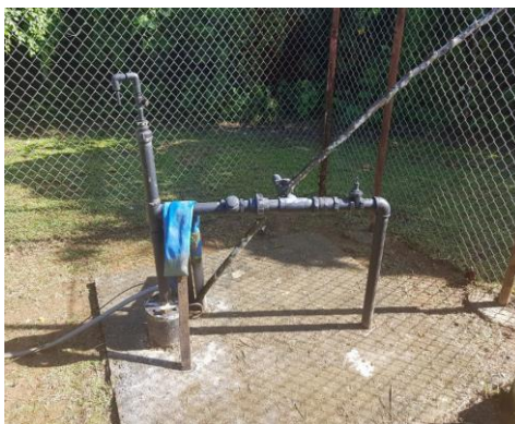
Fig 2 Example of well headwork to be replaced
