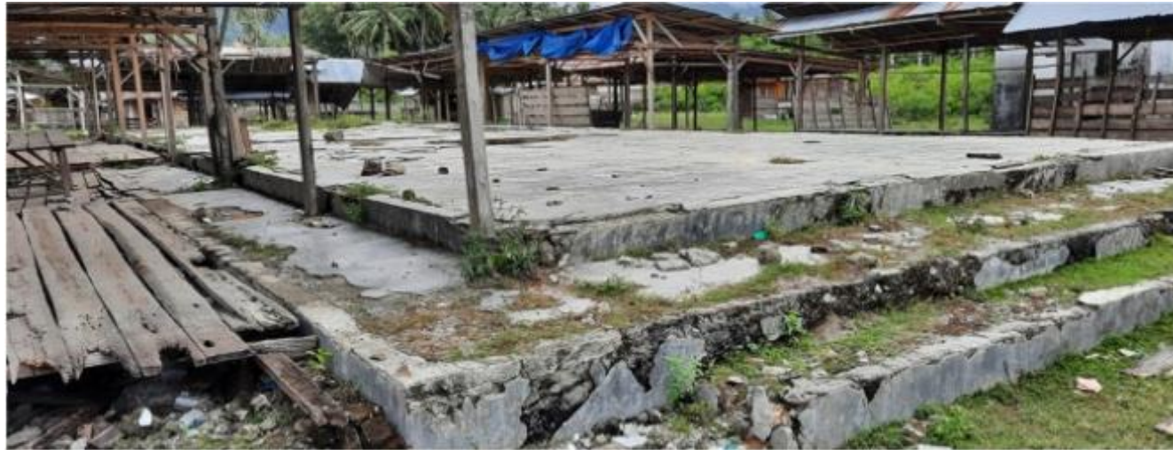
The condition of the existing booth was damaged by the earthquake
