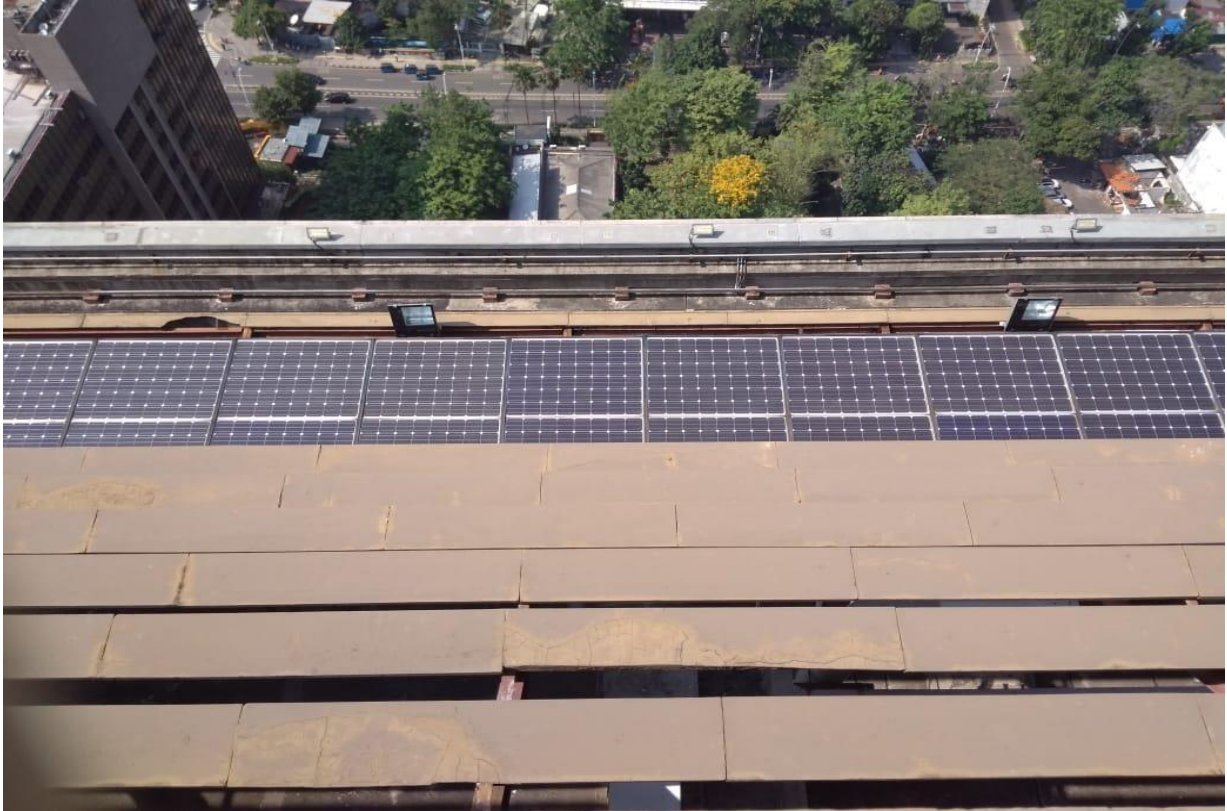
Figure 5-Images of existing 22 kWp Solar PV System
