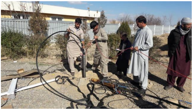
Pic 2: Installation in progress of a Solar Pump (Submersal) in a of a health facility in Herat (Source:
