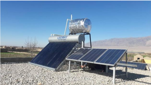
Pic 1: Solar water heater and solar PV panels installed on the roof of a health facility in Herat (Source: UNDP)
