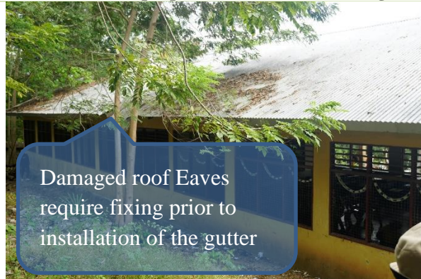
Small damaged on the roof eaves of the proposed building
