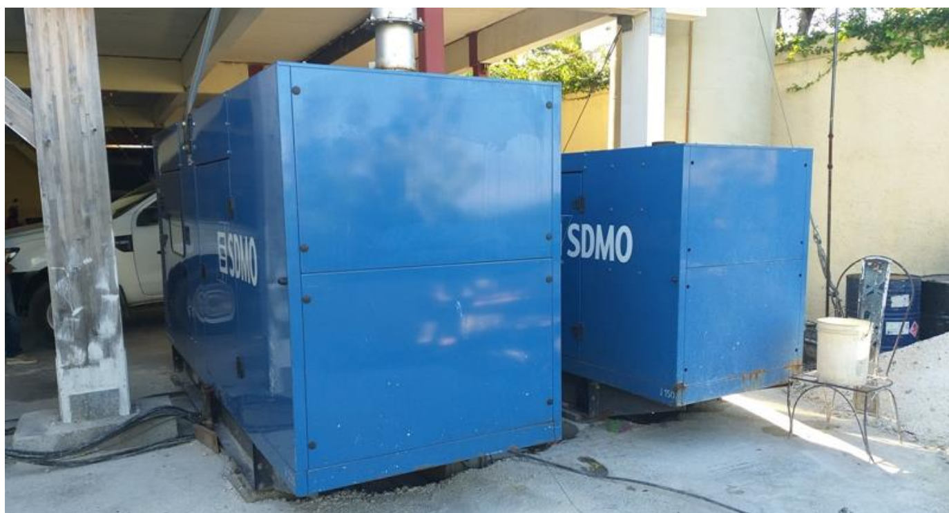
Figure 9 – Main and backup diesel generators
