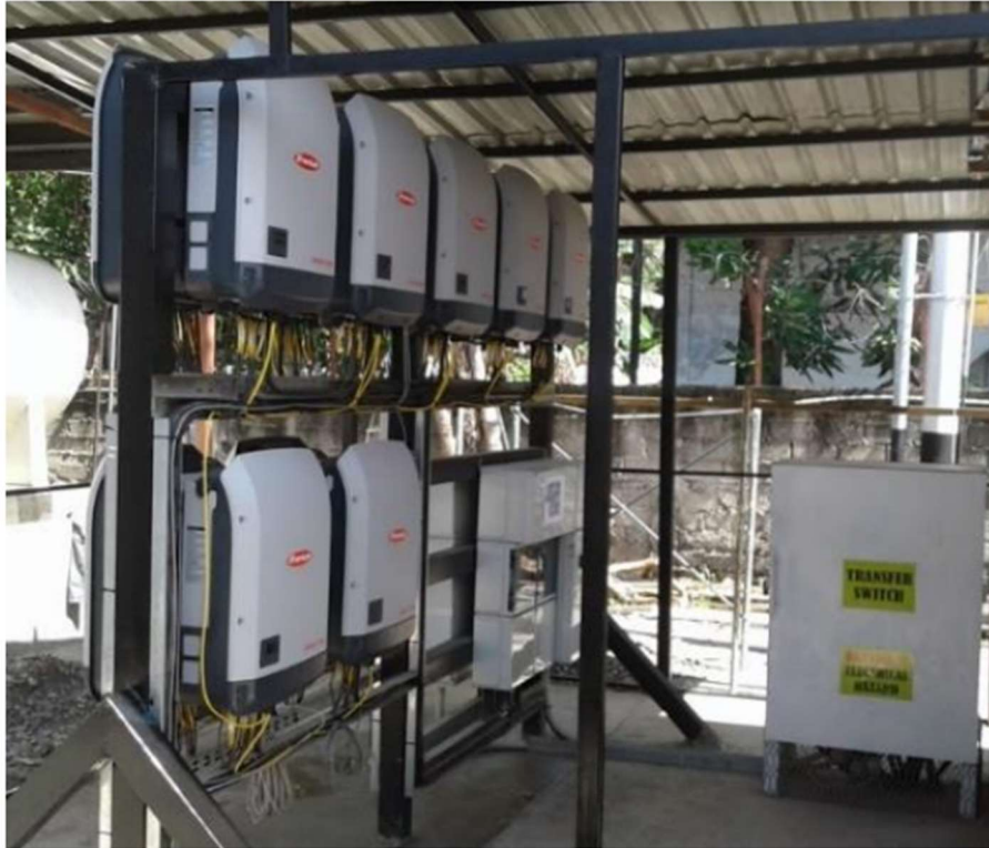
Figure 10: Inverter wall
