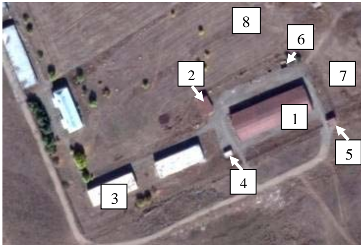
Picture 4. Structures to be designed and estimated in the scope of this assignment.
