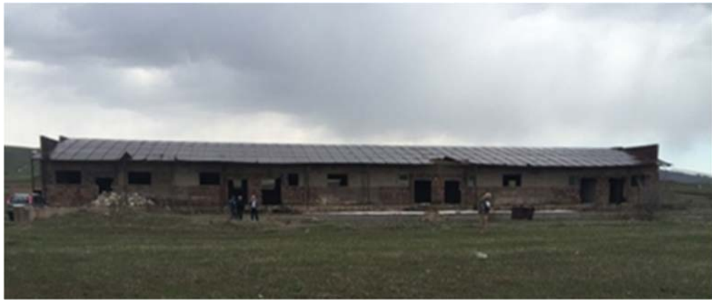
Picture 2. Main Storage Building
